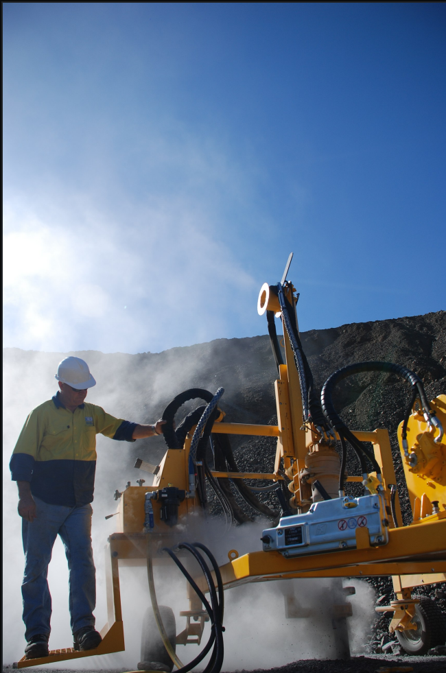
THE DRILLER AT THE CONTROLS WITH THE HOLE UNDER WAY
