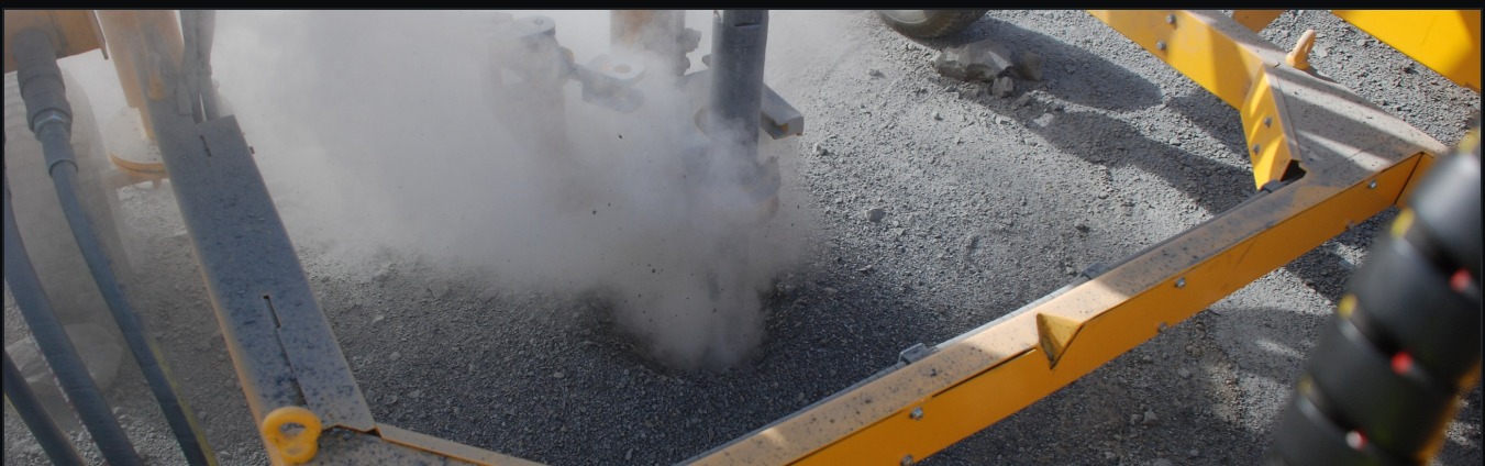
FLUSHING AT THE COLLAR – HOSES RUNNING BACK TO THE POWER PACK
