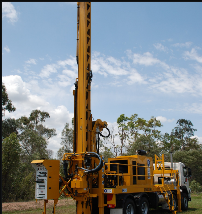
MAST ERECTED ON SITE, CONTROL PANEL SWUNG OUT TO THE DRILLER'S POSITION
