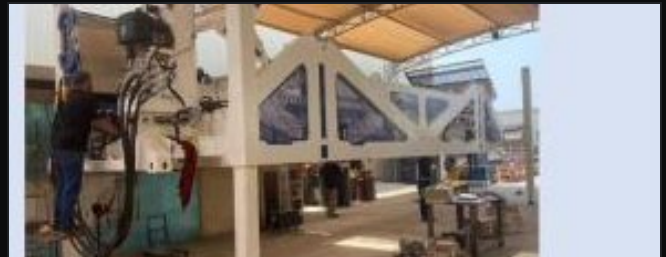
FABRICATION OF THE MAGAZINE FRAME
