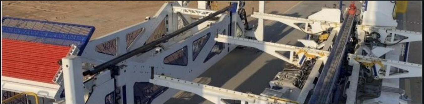
MAGAZINE ALIGNED TO THE CATWALK ON SITE
