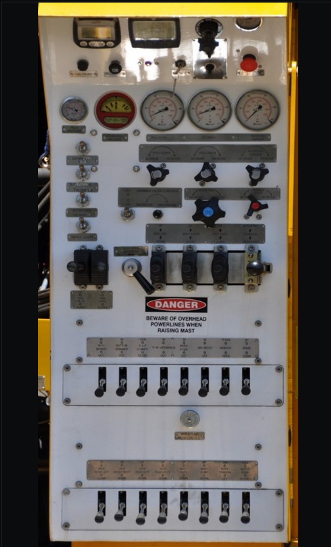
THE HYDRAULIC PIVOTING CONTROL PANEL
